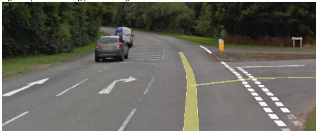
Fig3 Proposed crossing point looking south towards the Bourton Road roundabout.
