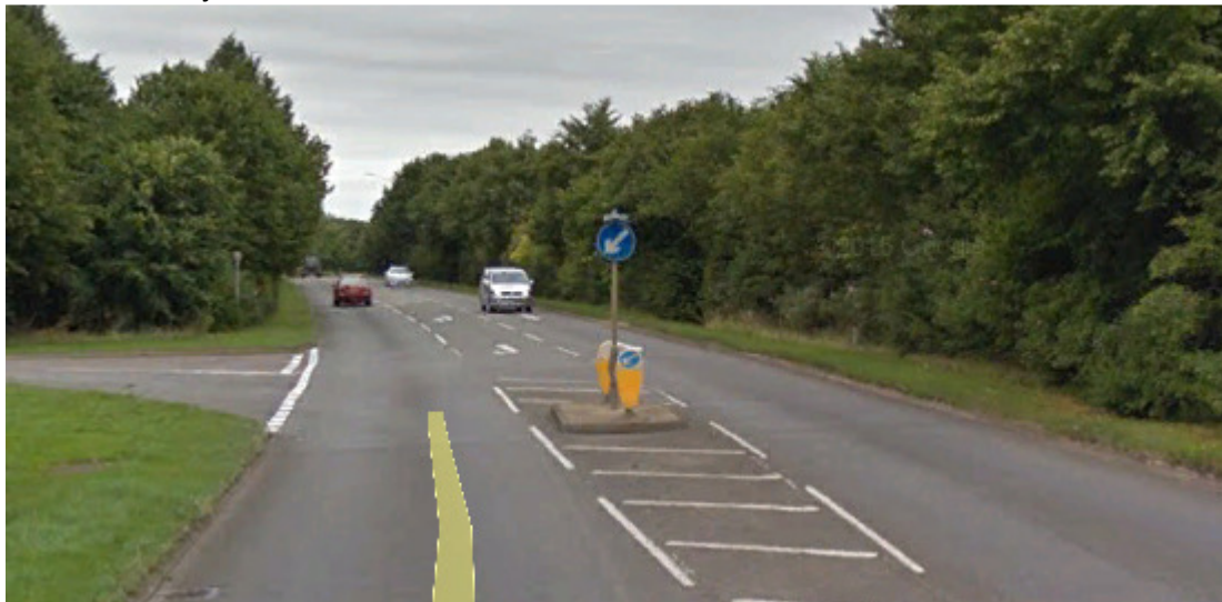
Fig5 Northern entrance to Linden Village does have a refuge. I am not sure why a refuge was installed at his junction but not at the southern entrance.
