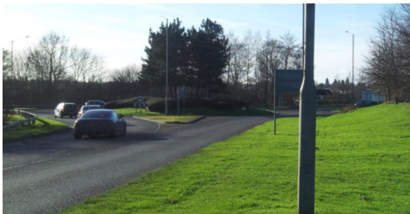
Fig2 View from MMT/5(BW)/1 path looking towards Buckingham town centre.
