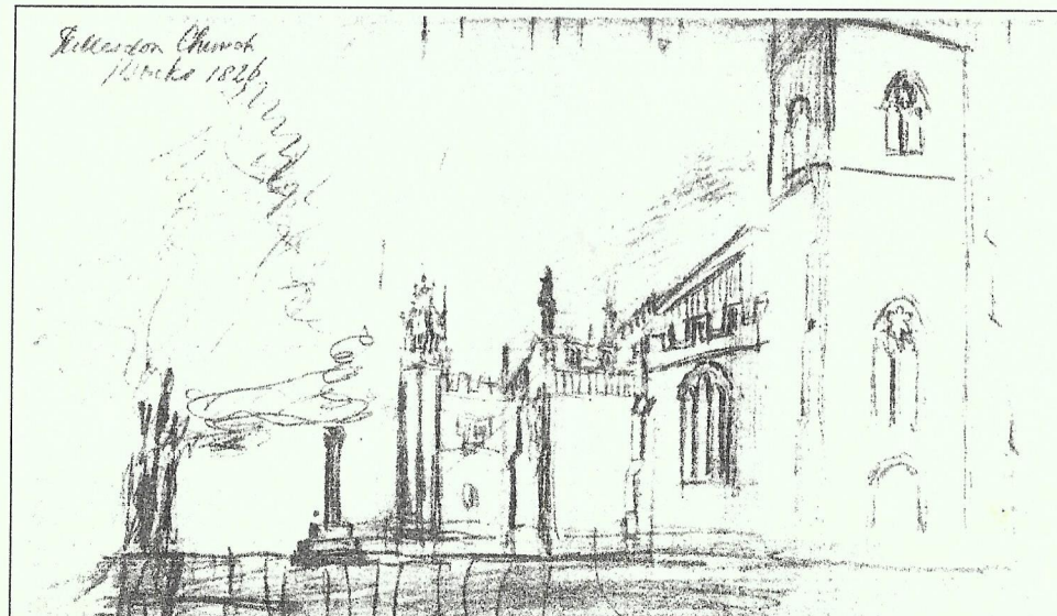
All Saints, Hillesden , sketched by George Gilbert Scott aged 15, around the time that Revd Thomas Scott asked the Duke of Buckingham to repair it. His response to whitewash the exterior of the tower - an act of inappropriate restoration!
